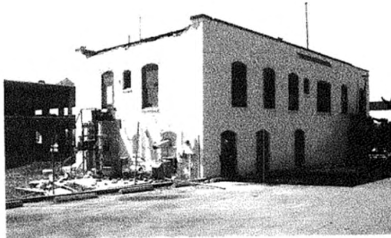
Figure 6-5 Unreinforced masonry wall with a stepped crack.
