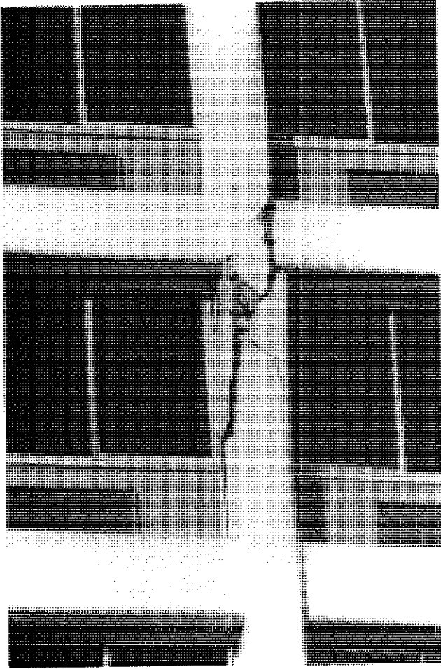
Figure 8-5 Close-up of fractured column. This column lacks confinement of its vertical reinforcement and has essentially lost its capacity to carry vertical loads. Post Unsafe.
