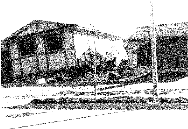
Condition 1: Collapse, partial collapse, or moved off foundation. Post Unsafe.
