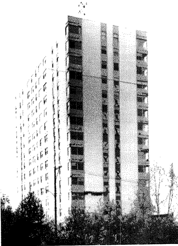
Figure 8-11 Shear-wall failure from 1964 Alaska earthquake. Post similarly damaged structures Unsafe.
