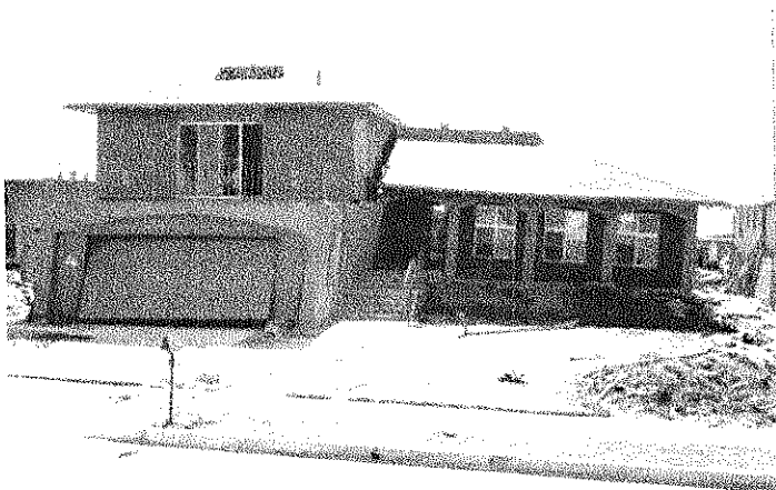
Figure 5-2 There is residual lean in the garage opening and separation between portions of the structure. Post Unsafe.
