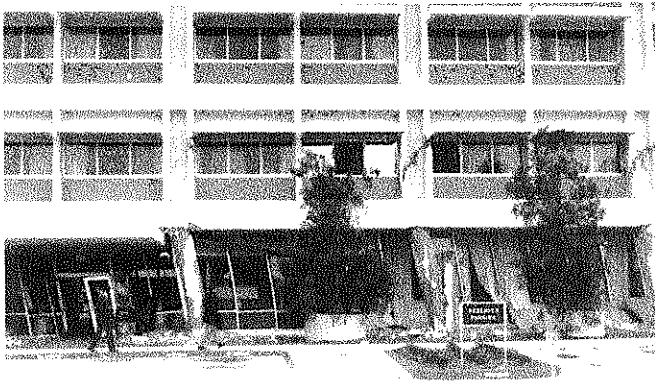
Condition 1: Collapse, partial collapse, or moved off foundation. Post Unsafe.
