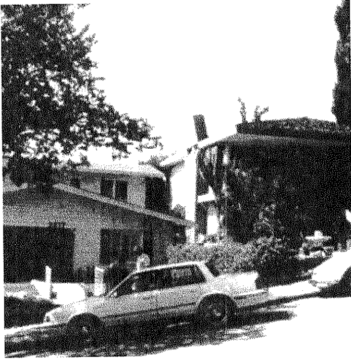
Figure E-10 The home with the leaning chimney from Example 3 is shown on the right.
