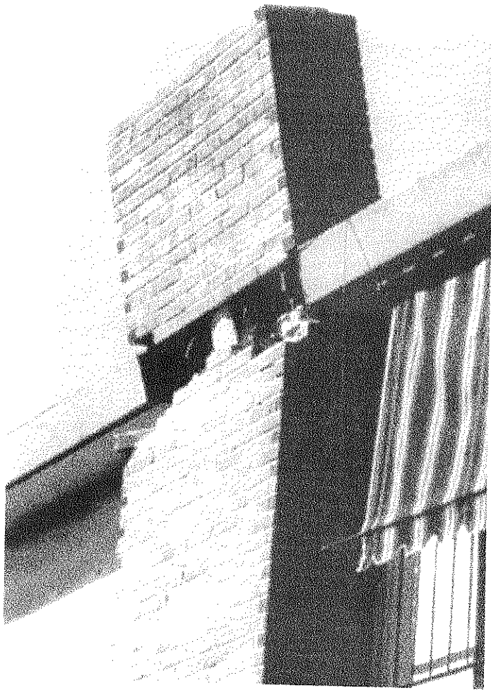
Figure E-11 This leaning chimney from Example 3 has been severely damaged and presents a serious falling hazard. (Note: In some cases, chimneys may be in danger of falling through the roof into the dwelling. In such cases, interior spaces should be barricaded.)
